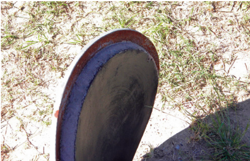
TEMPORARY ACCESS CLOSURE COMPLETE WITH INTERNAL CORROSION PROTECTION
