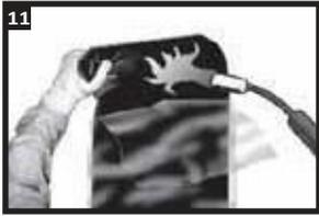
Partially remove the release liner and gently heat the underlap approximately 150mm (6") from the edge.
