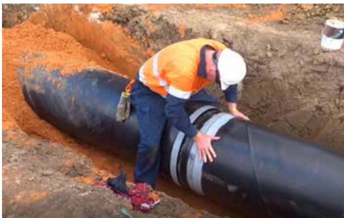
Sintalock I - Rubber Ring Joint
